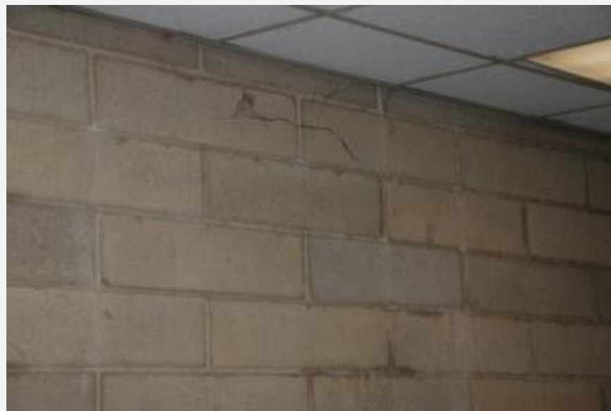
Cracked masonry
