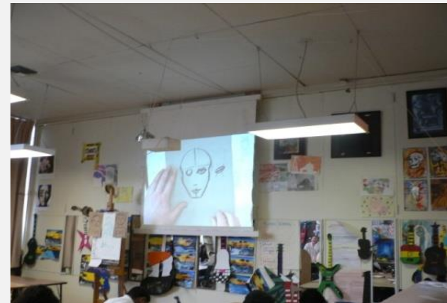
Improper suspension / bracing of equipment
