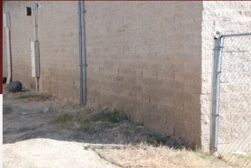
Landscaping and earth above finish floor level
