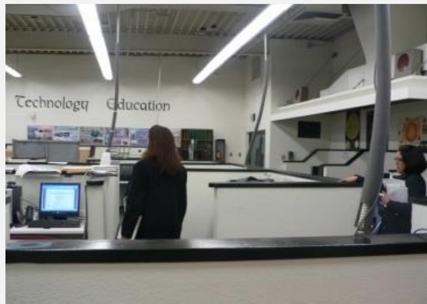
Non-code compliant wiring
