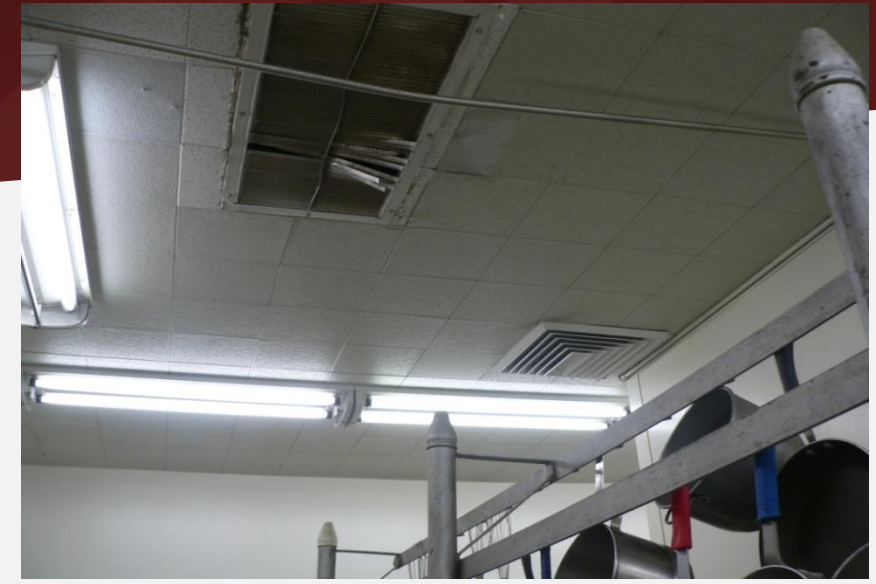
Vent at existing kitchen
