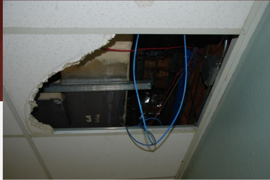
Existing ceiling conditions
