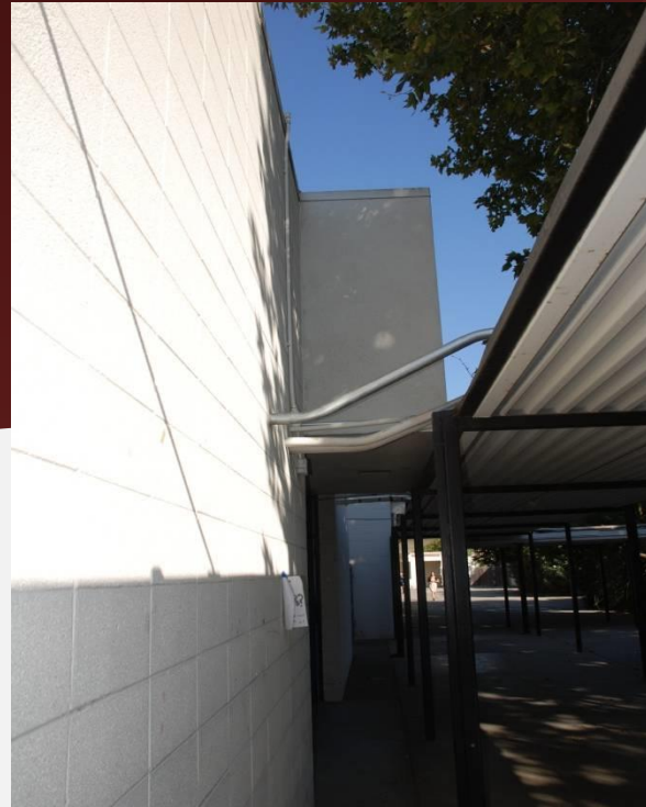
Rigid connection between separate structures
