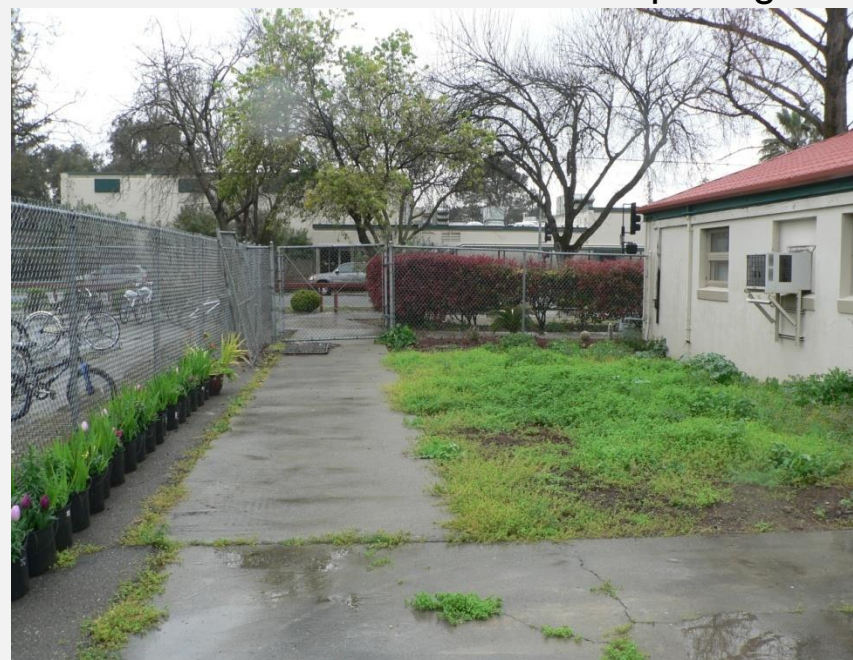
Deteriorated inefficient landscaping
