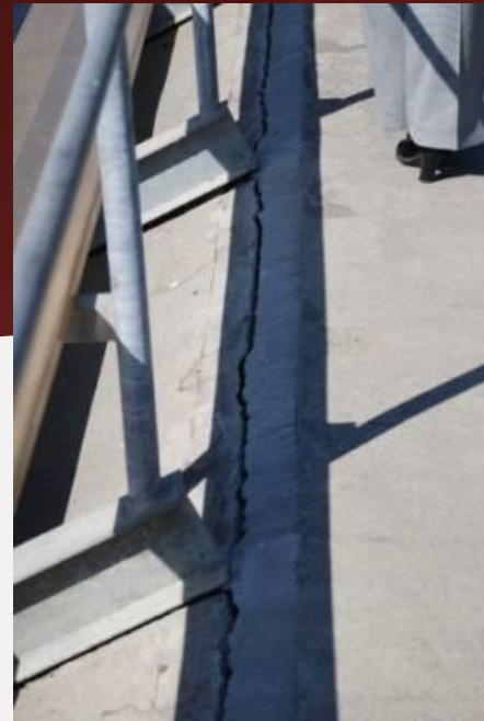
Cracked concrete at stadium
