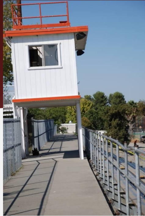
Settlement at existing press box
